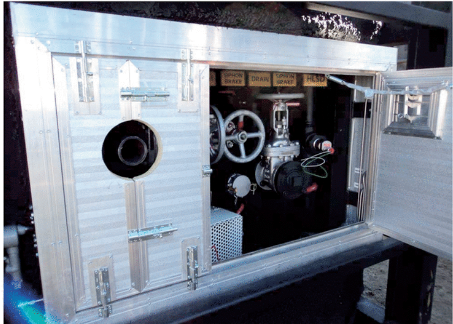
Top: The DuoVault contains all the valves and connections within the outer tank, creating a true double-wall design, say company officials.
